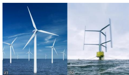
Fig. 0.2. Classification of turbines based on the turbine axis position
