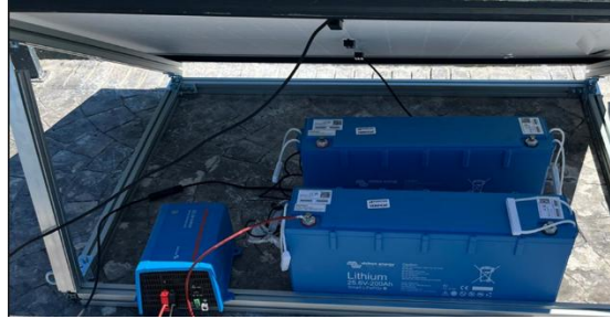
Figure 5.21 – LiFePO4 batteries and inverter used in the project
