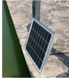
Figure 5.1 – Photovoltaic panel with a power of 10Wp mounted on the lakeshore – SPMS Palazu-Mare
