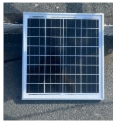
Figure 5.9 – Mounting the photovoltaic panel on a surface covered with bitumen/pitch
