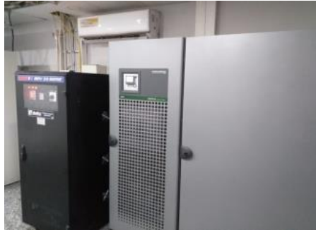
Figure 4.3. The 150 kVA UPS and Automatic Voltage Regulators located in Technical Room.
